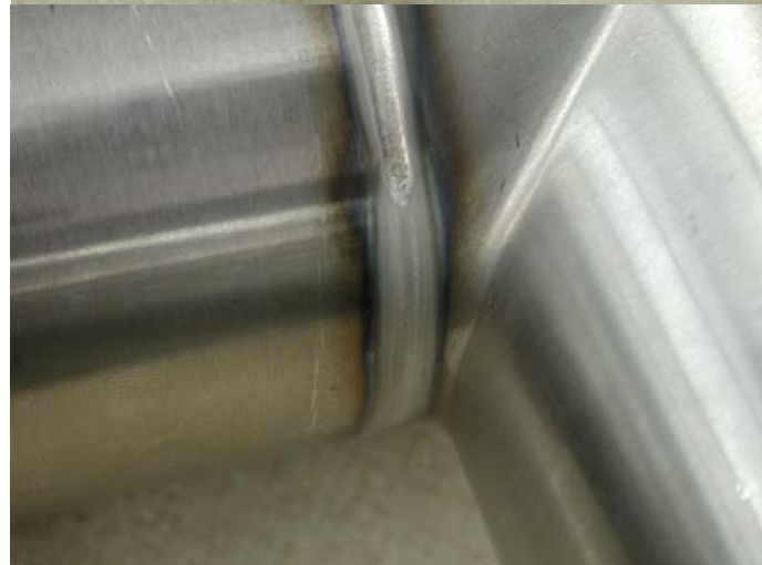
Close up view of completed weld joint.
