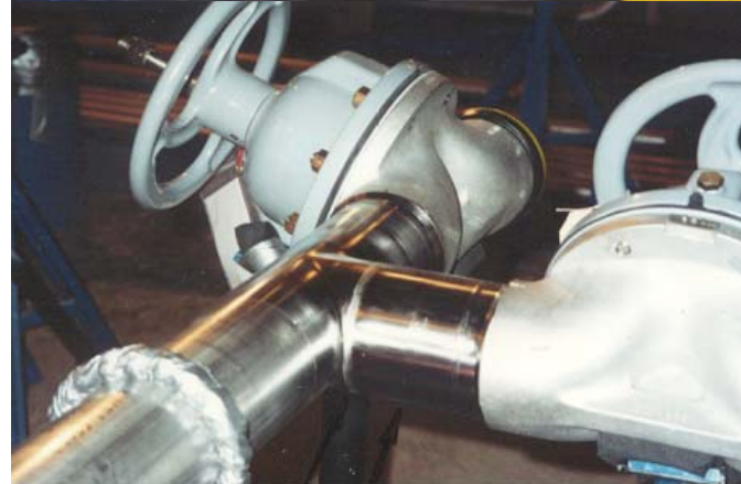
Field Welded Joint
